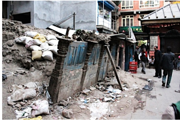
6. Crumbling medieval buildings and modern concrete homes.
