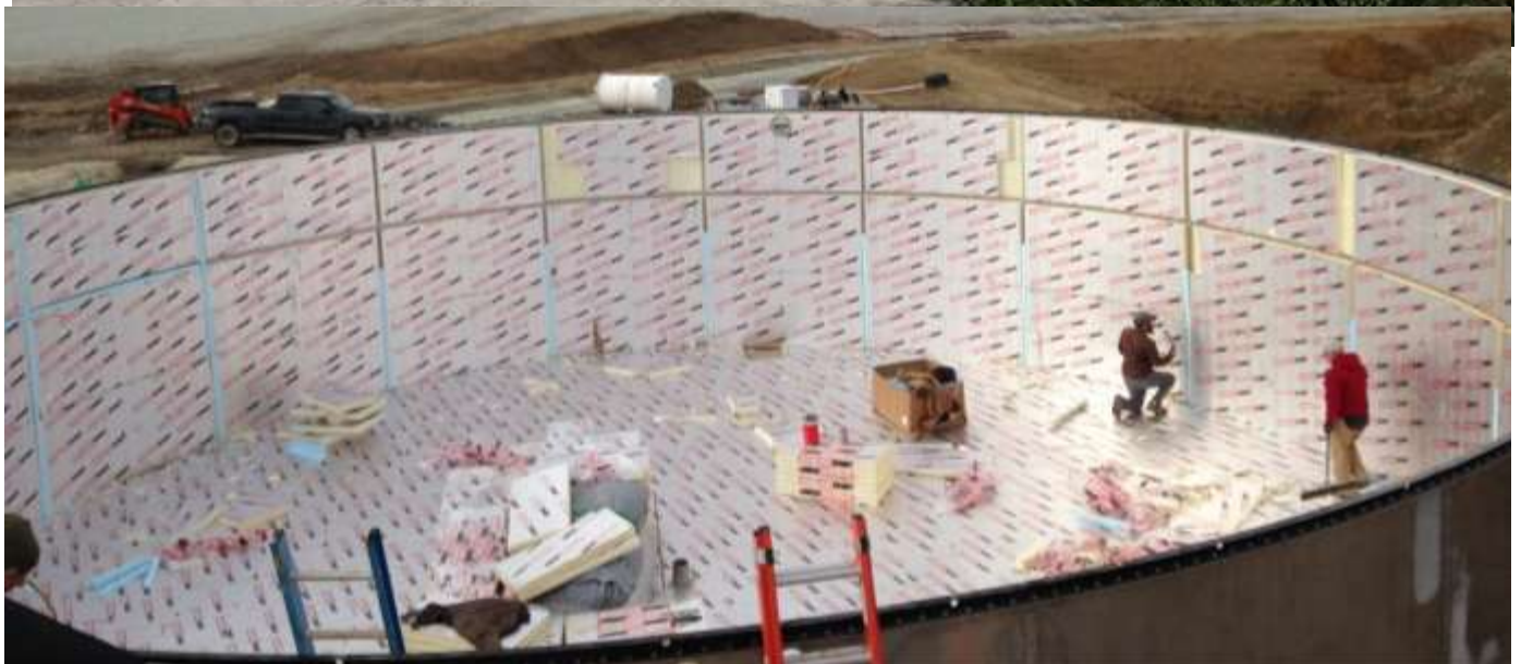
The mini digester package is a kit designed for quick installation (1-2 weeks or less). After a system is sized to meet feedstock loading volume and owner goals, a concrete pad is poured
